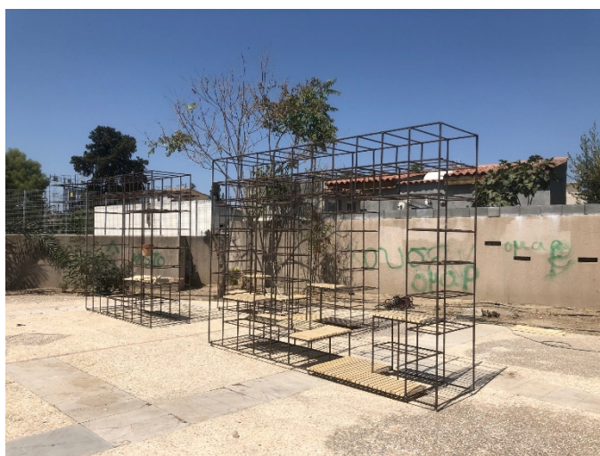
Figure 13. The steel structure was used as a participatory open framework for engagement. Source: Urban Gorillas
