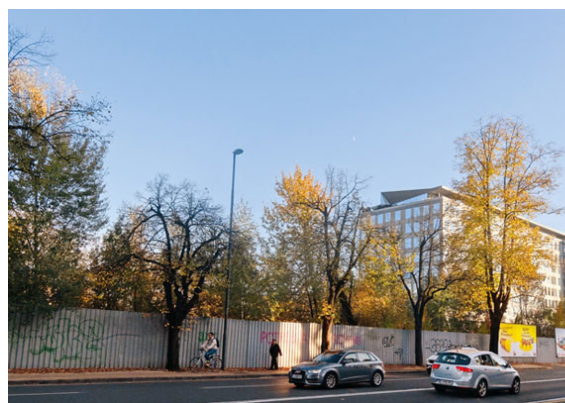
Figure 2. A hidden place behind the construction fence – view from the street
